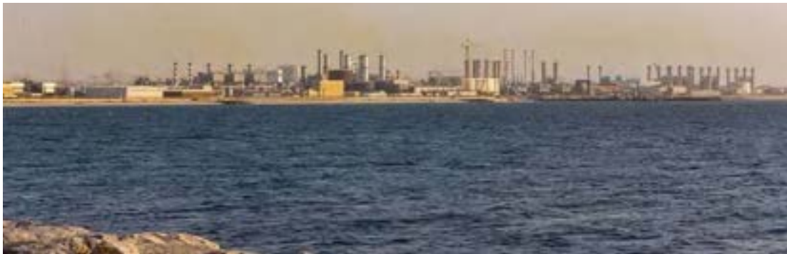
Power and desalination plant in Dubai
